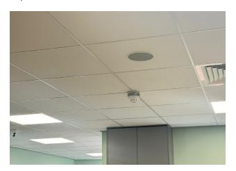
In the canteen area we also specified the PC-1860 ceiling speakers again connected to an A-2120DD amplifier with an IP-A1AF IP Audio Interface and IP-A1PG IP Paging Gateway. In addition, this area also had installed the WS-5325H UHF wireless system with WH-4000H headset for local and full-facility broadcasts.
